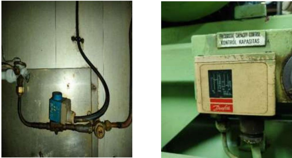
Gambar 3.2.1. *soloid Valves & Pressure Control*
